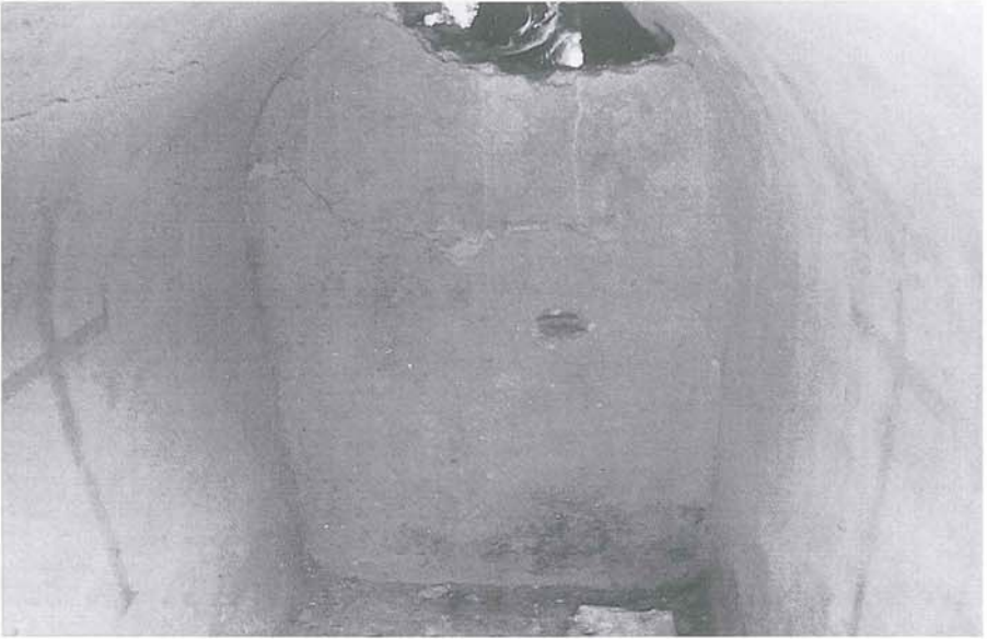
Figure 7. Between Silivrikapı and Mevlevihanekapı: interior of the hypogeum.
